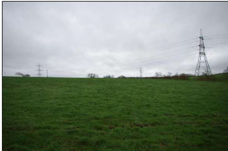
14. F2, VIEW ACROSS THE SURVEY AREA; VIEWED FROM THE NORTH-EAST (NO SCALE).
